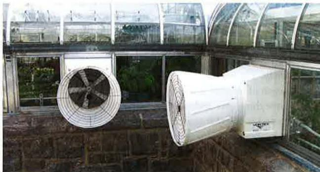
Adding a discharge cone to a fan provides at least 15 percent increased airflow.
