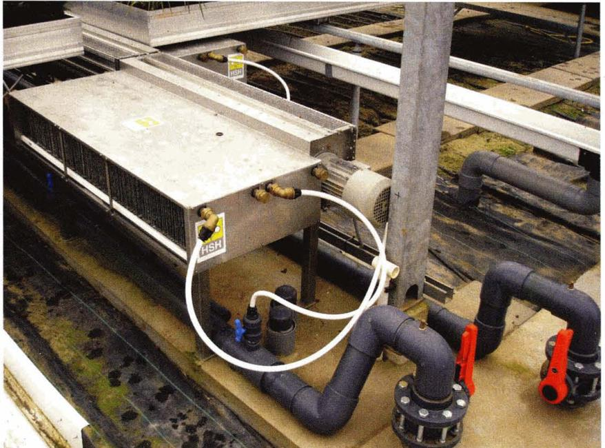
**FiWiHex heat exchangers use extremely thin copper tubes through which water flows and transfers energy. In the summer, the heat of the hot air exchanges with cool water in the tubes, cooling the greenhouse temperature and heating the water for the warm aquifer. The Dutch inventor asserts that FiWiHex can decrease natural gas usage 5 to 10 meters<sup>3</sup> per meter<sup>2</sup> of greenhouse space.**
